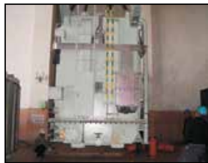
35kV steel Furnace Plant installation
