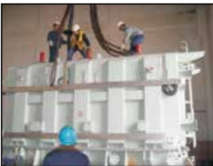
220kV Steel plant installation
